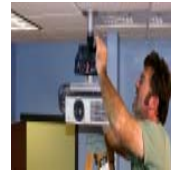
Pole Mount Platform Installation
